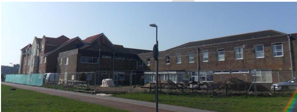
Cherry Garth Elderly Persons' Home transforming in a two-phase build process into Meadowfields Extra Care
